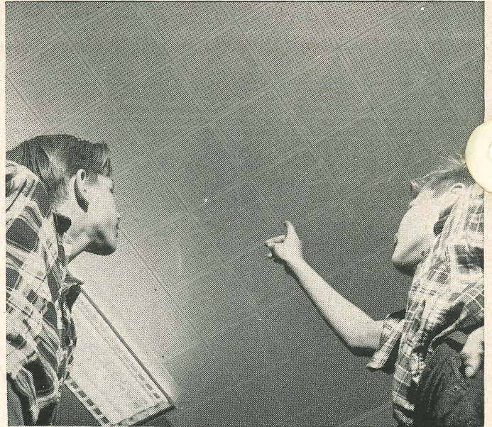
FROM FLOOR COVERING the boys' attention went to the new "Acousticfibre" ceiling with its myriads of little perforations necessary to remove echoes and noises which are so detrimental to the efficient performance of our "Trainear" equipment.
