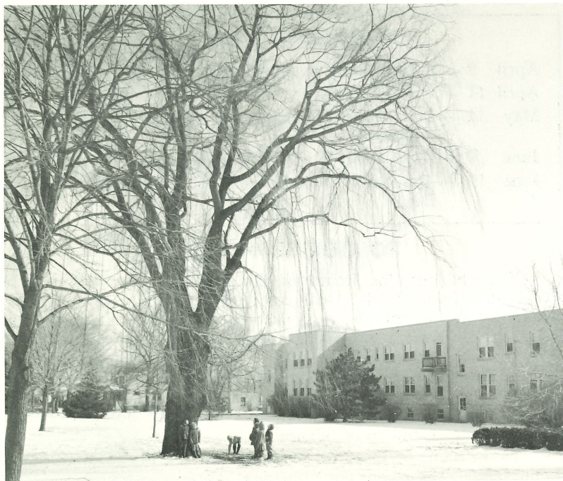
A group of our little boys looking at the tremendous size of the "Big Willow" which stands directly in the new building wing area.
