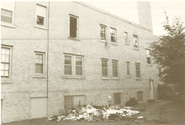
The remains of the linen storage room
